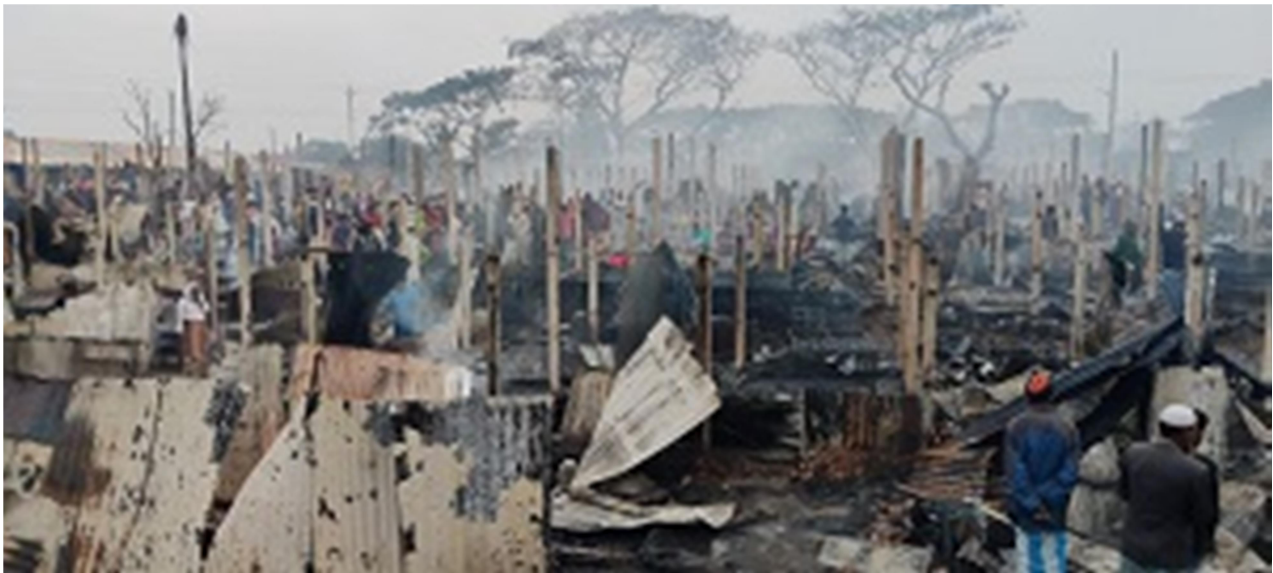
Picture-1 showing huge damages as a result of fire outbreak at the midnight on 15 January 2021
